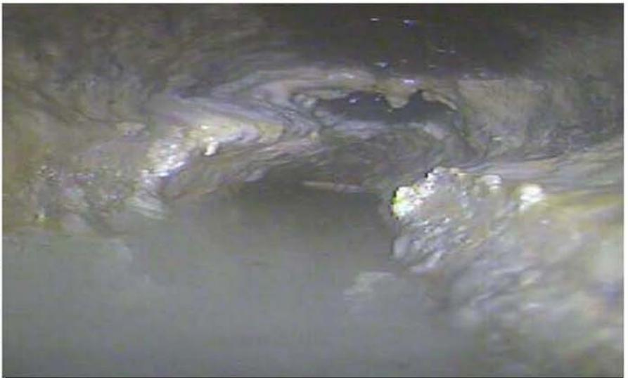
This 4-inch lateral line is reduced to less than 2-inches in diameter because of grease!
